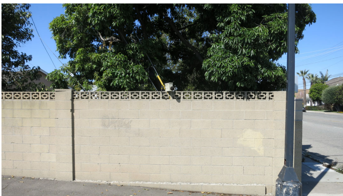
Noise Measurement Site L1 - looking west
