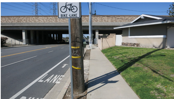
Noise Measurement Site L3 - looking west
