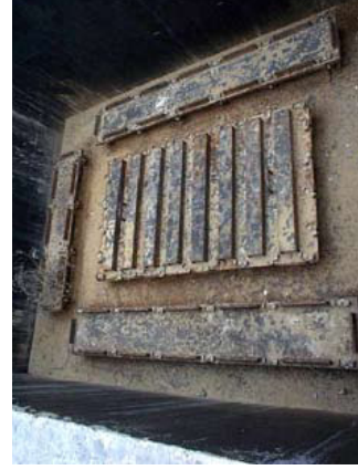
2 Junction Box (STA 19+29) and Transition Structure No. 1
