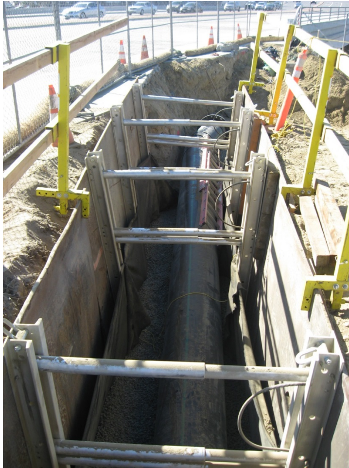
Figure 2.5-2: Typical Open-Cut Trench Shoring
