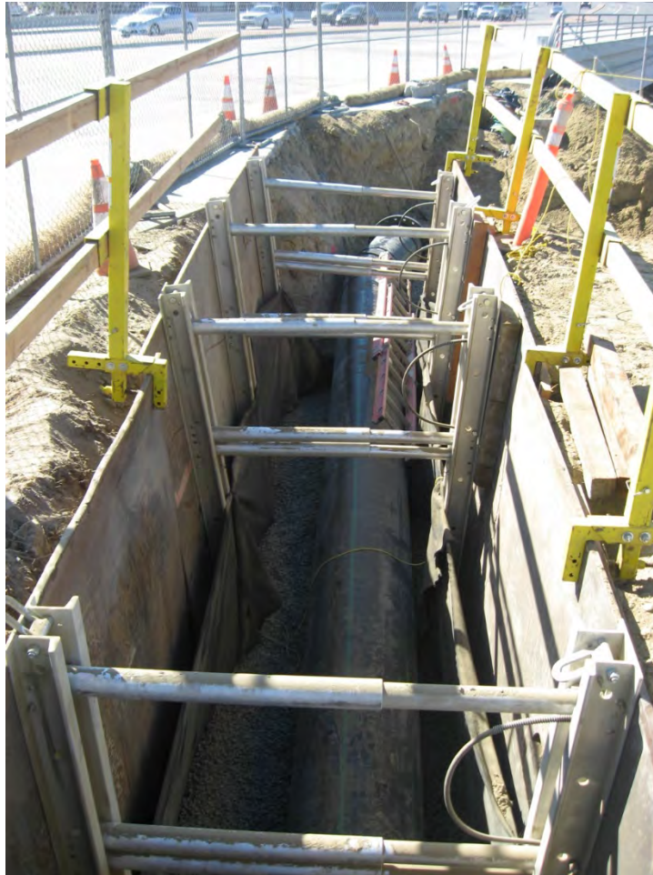
Figure 2.5-2: Typical Open-Cut Trench Shoring
