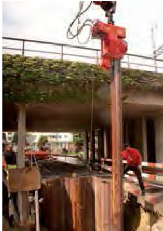
Figure 2.4-2: Westside Pump Station Shoring – Typical Vibratory Pile Driving Method
